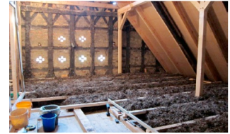
Figure 9 Seagrass roof insulation
